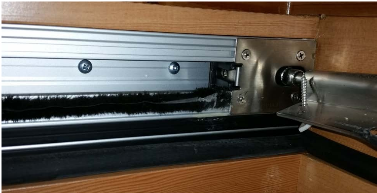
Head Track with Pile Weather-stripping
