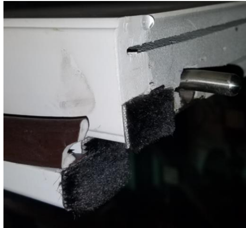
Astragal with pile dust pads
