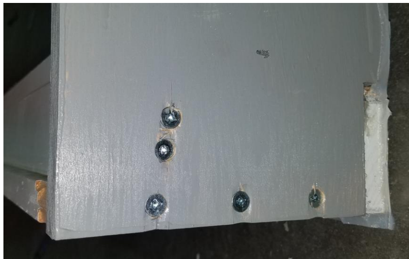
Corner joint screws at the head
