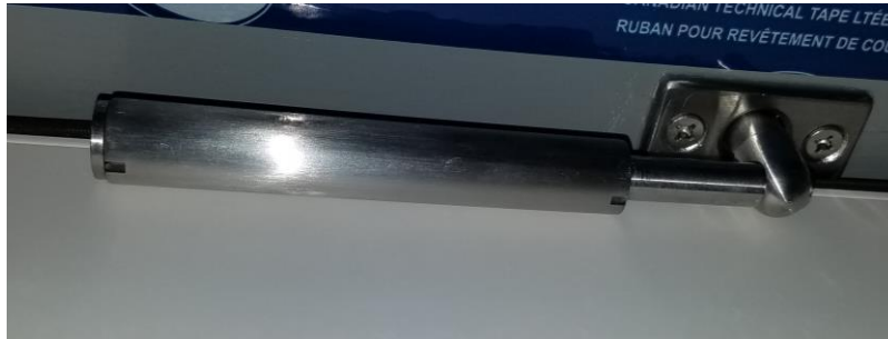
Mid-point hinge at the jamb
