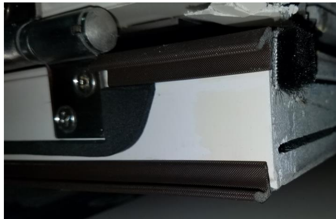
Door panel stile weather-stripping configuration
