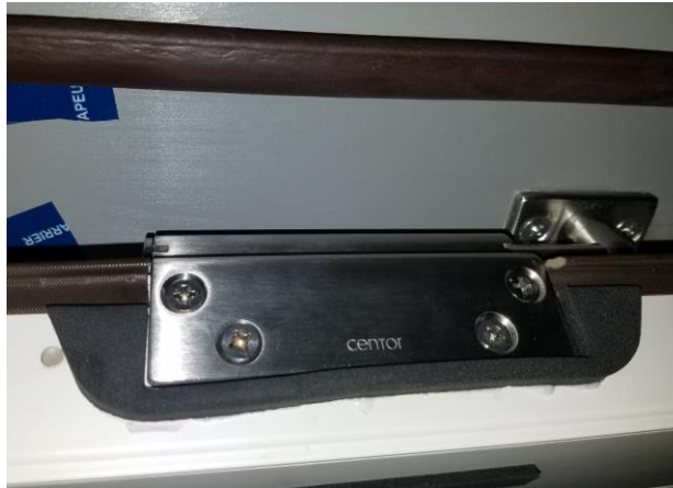
C-shaped gasket around the hinge locations
