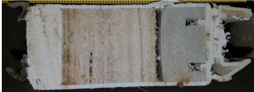
Panel 2 right side stile (from exterior)
