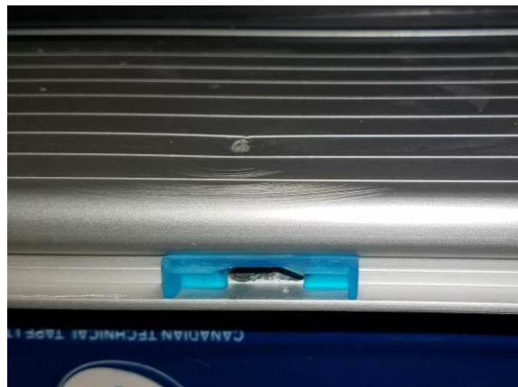
Drain slot out from the sill with drain cover
