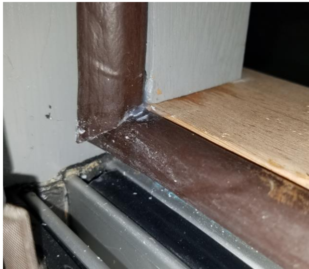
Frame weather-stripping corner
